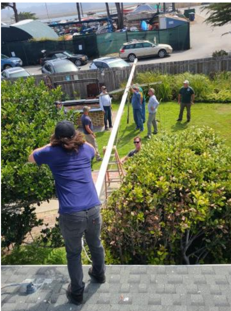
Mast restoration A team of volunteers lowered the club mast for needed repairs.
